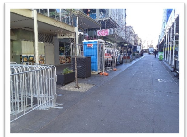
Bank Street After Photo 4.
